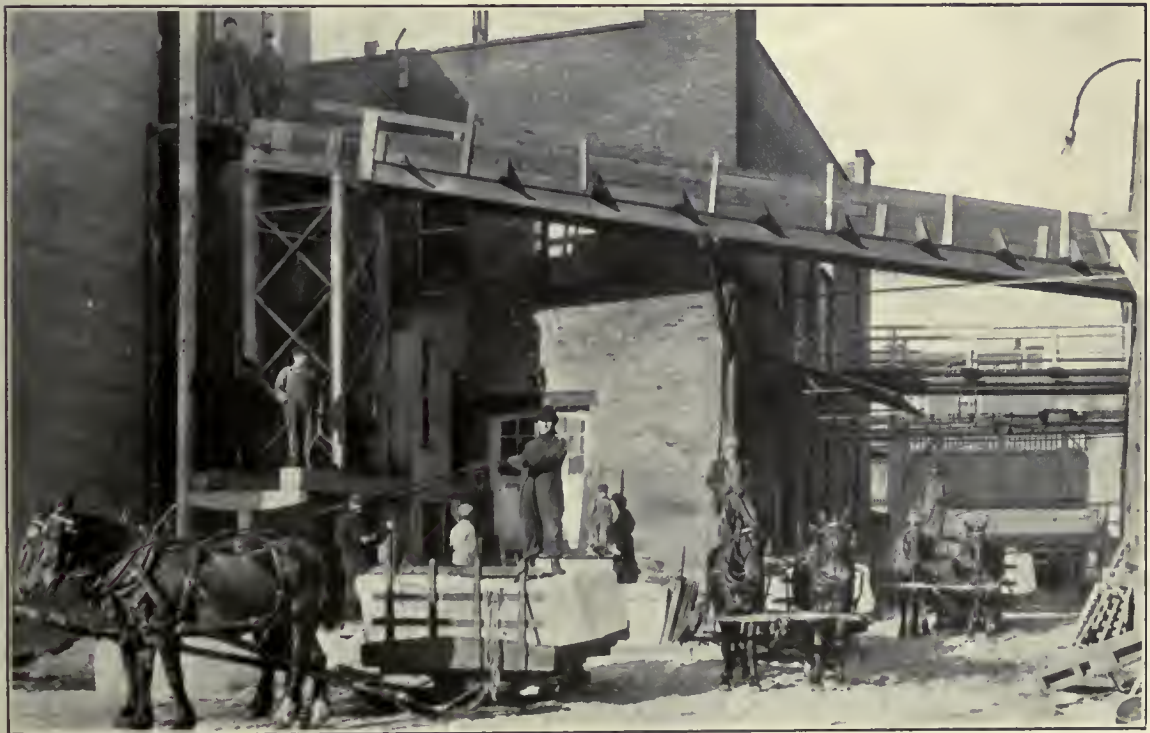
ICE HOUSE OF THE MONTREAL DAIRY CO., LIMITED. Capacity 7,000 tons.
